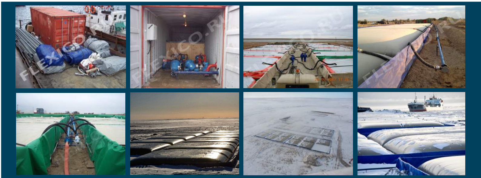
FIELD FUEL STORAGE UNIT WITH NOMINAL CAPACITY OF 1000 M3 IS MOUNTING FOR 3 DAYS BY 8 PERSONS!
